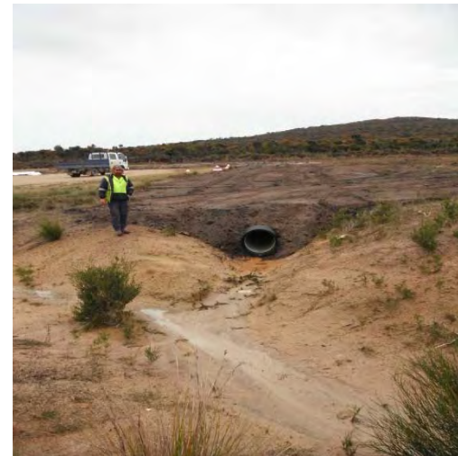
Runway End Drainage after
