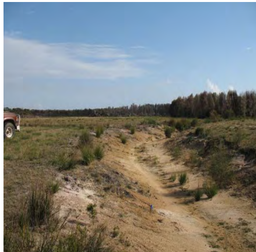
Runway End Drainage before
